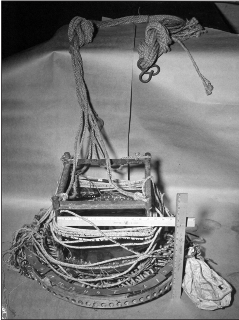
The altitude control mechanism (left) and two sandbags recovered from the Japanese balloon that landed near the lower Yukon River community of Marshall on December 23, 1944. Note the empty sandbag attached to the control mechanism. Photographs courtesy of the National Archives and Records Administration, College Park, Maryland. (Box 42, RG 499)
