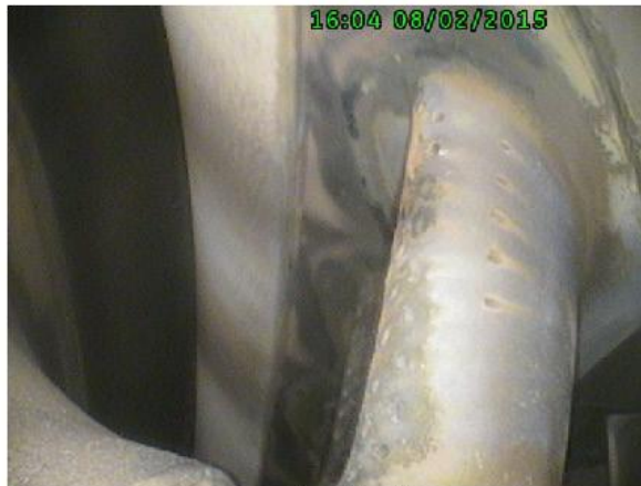
Photo No. 11 High pressure turbine vane ring.
