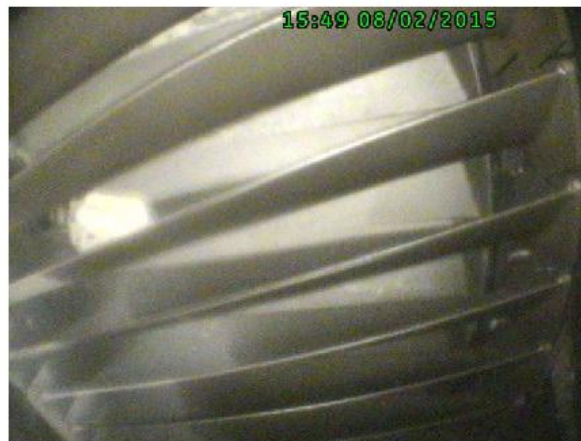
Photo No. 7 First stage power turbine.
