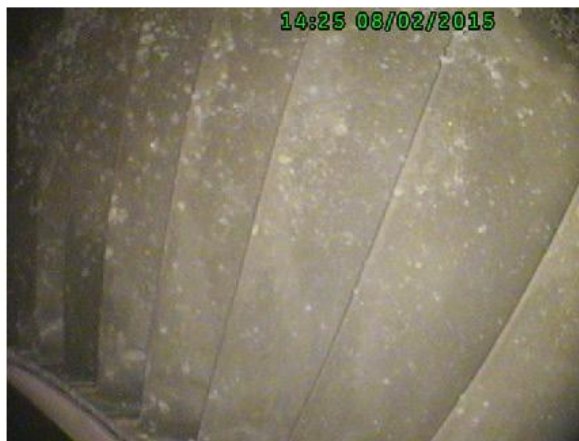
Photo No. 38 Second stage power turbine.
